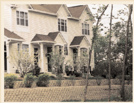
Fisher Burton built this attractive retaining wall of buff-colored Anchor Diamond® beveled blocks to enhance the landscape surrounding a new housing development in suburban Chicago.
