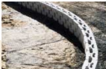
Miragrid™ polyester geogrids serve as the soil reinforcement elements to strengthen and stabilize the Anchor Vertica® wall.
