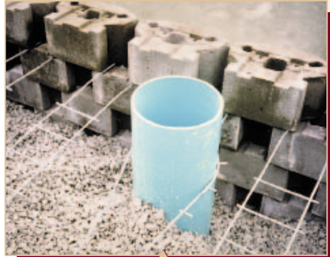
Detail at Intersection of Vertical Post Form and Keystrip Steel Reinforcement
