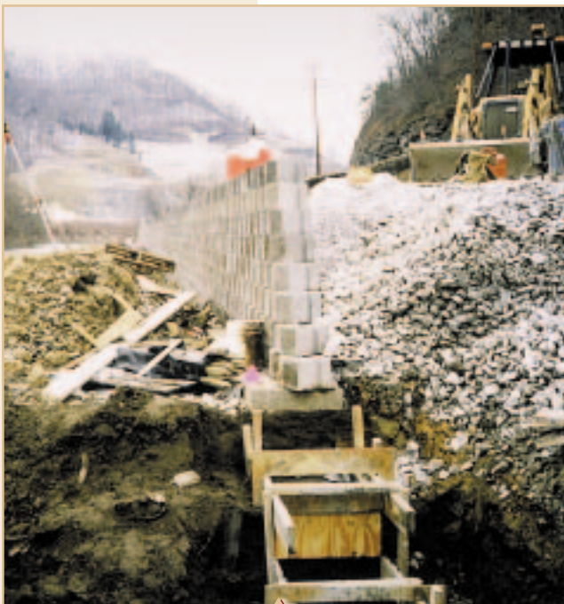
Partial Wall Shown with Forming for Additional Concrete Leveling Pad
