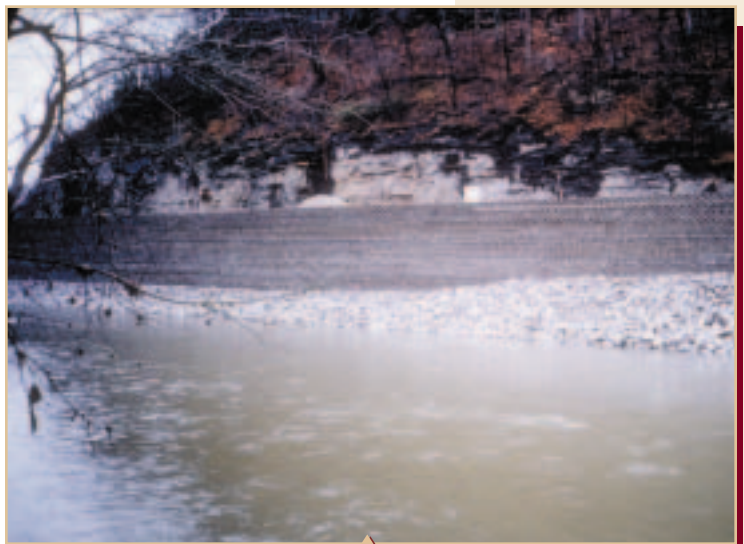
View from opposite shore of the Keystone Flood wall on the Cumberland River
