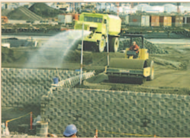
Select Granular Fill With Vibratory Compaction
