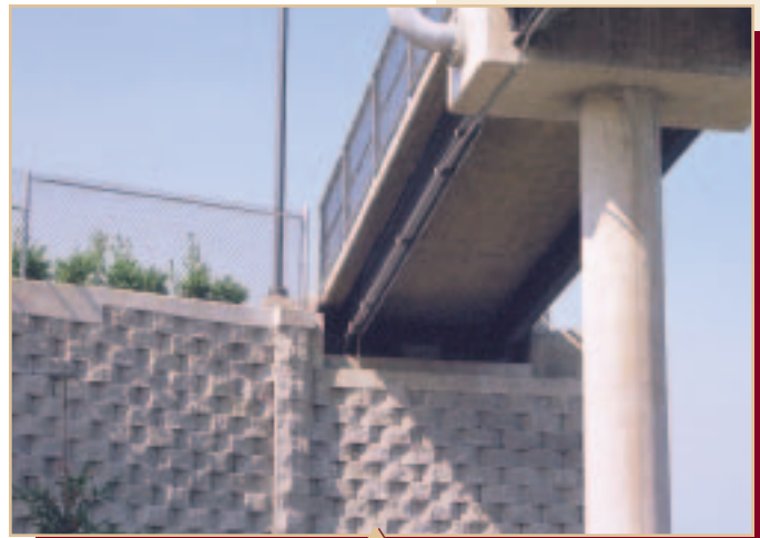
Pedestrian Bridge Supported By "Near Vertical" Keystone Wall
