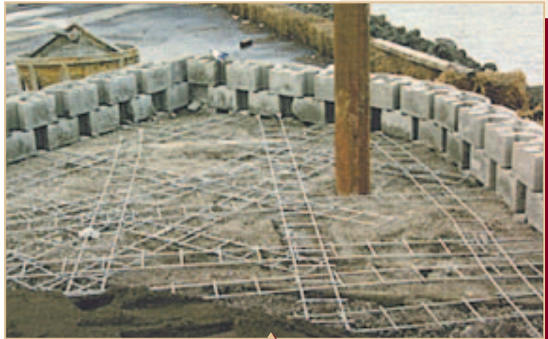
Steel Reinforcing Layout at Bridge Support Point
