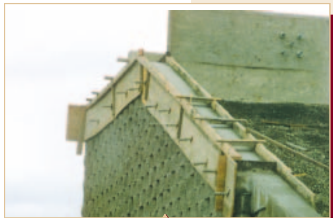
Forming of Site Poured Copings
