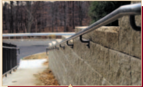
Pedestrian ramp with handrail detailed
