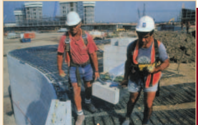
Construction continues with Keystone and geogrid
