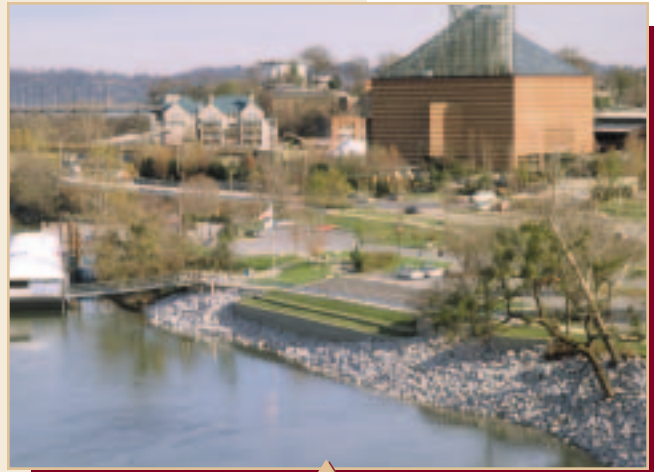
Retaining Wall Solution Protects Park Area
