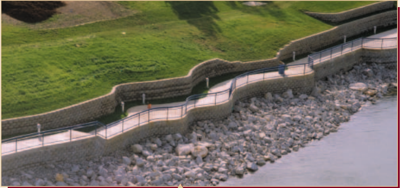
Flood Protection and Pedestrian Riverwalk come together at Historic Riverfront
