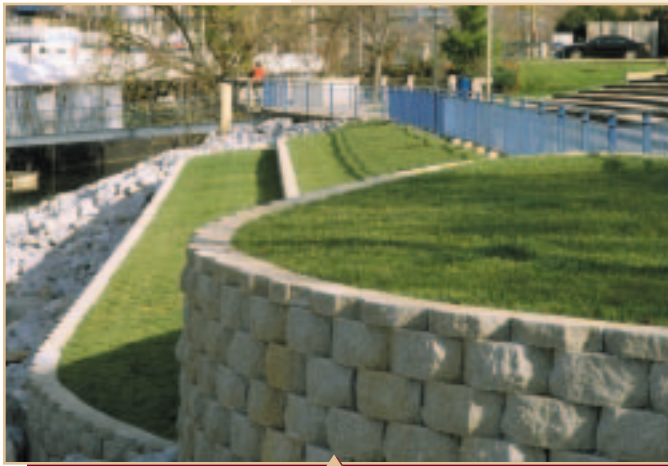
New Terrace wall protects amphitheater from erosion
