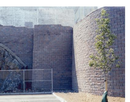
while offering a natural stone look and feel to complement the existing environment. The Keystone Compac wall was also less expensive than a poured-in-place wall and more durable than a timber wall.
