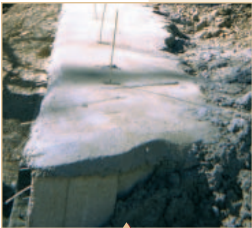
View of top of wall elevation showing grouted cap serving two purposes: (1) seal off water (2) secure wire to units and provide clean surface for rock attachment.
