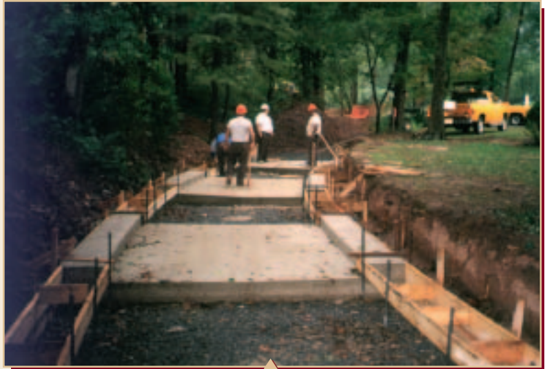
The Keystone units were placed on a concrete footing.
