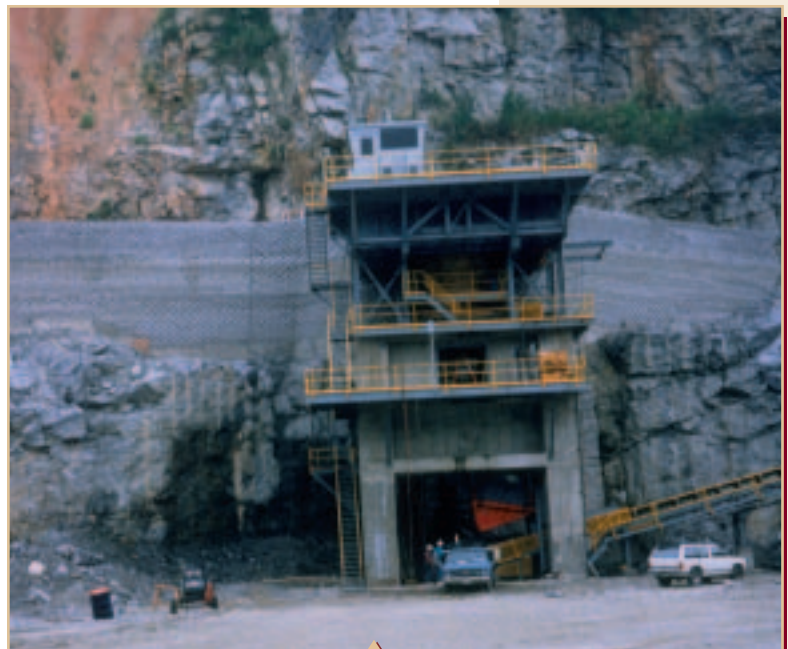
Rock quarry loading platform held with the Keystone Retaining Wall System
