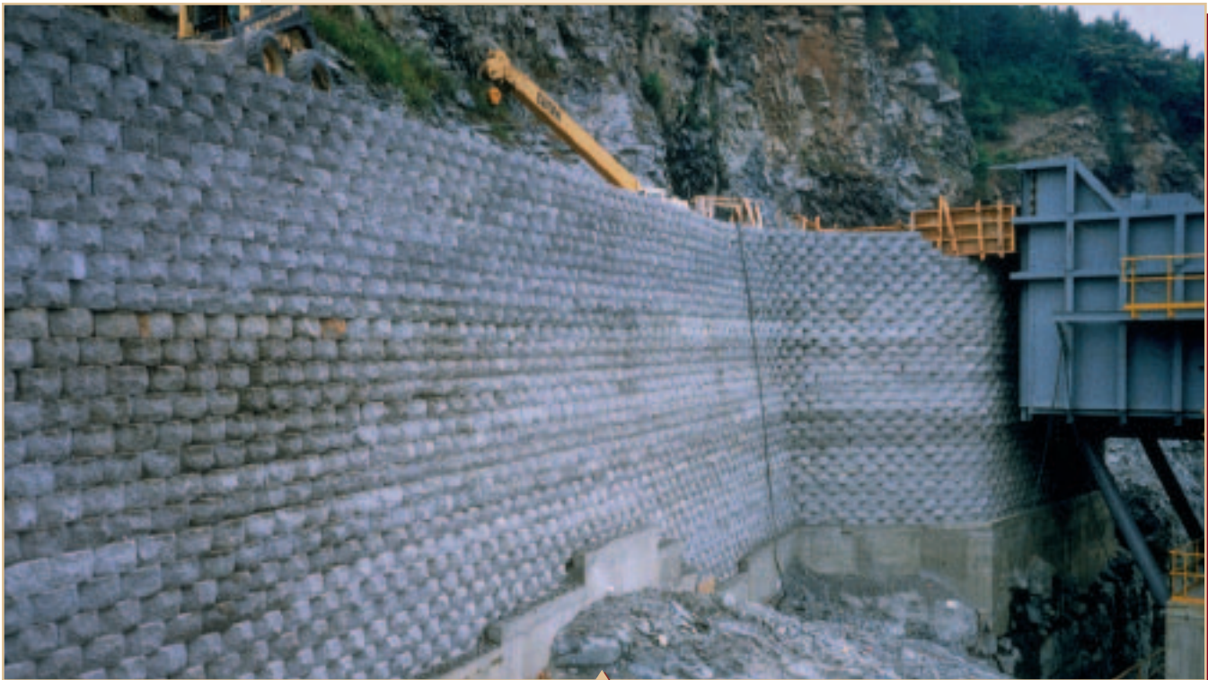
Keystone wall constructed on a reinforced concrete footing.
