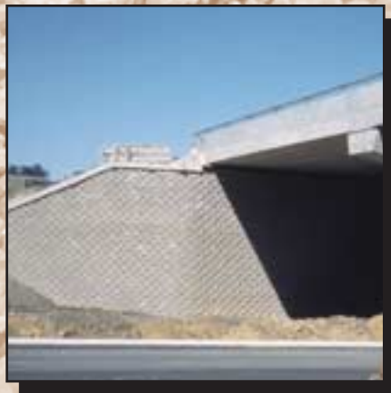
Alport, New Zealand bridge support and approach walls
