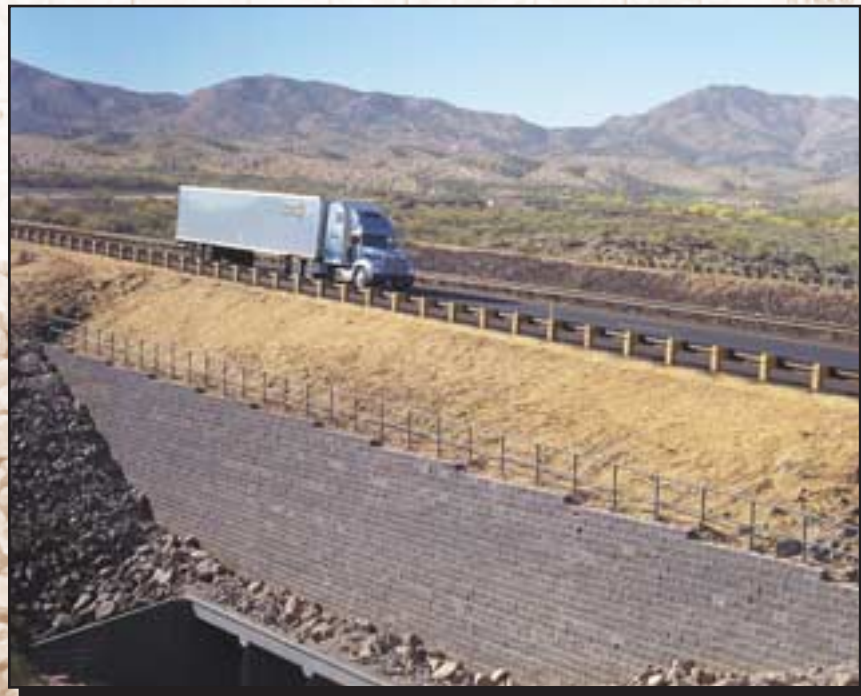
Wickenburg, Arizona - highway wall over drainage structure box culvert
