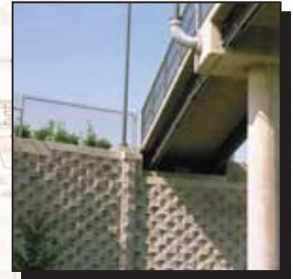
Bridge support and slip joint
