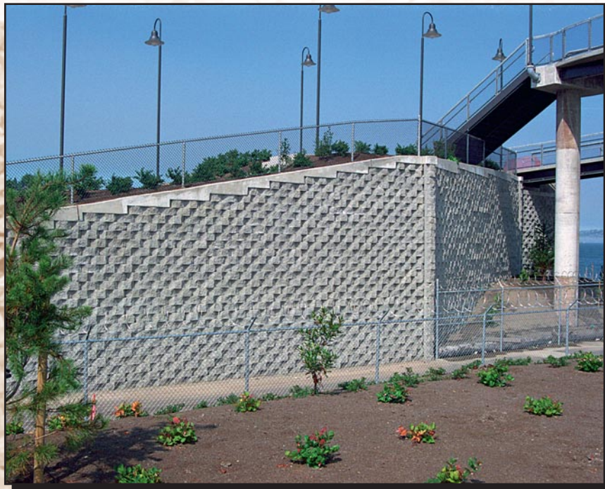
Terminal 5 - Seattle, Washington project
