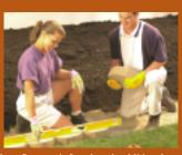
Place and level the first Sedona Stone unit. Level each additional unit on the base course as you place it, making sure that the side edges touch. If your wall contains both straight and curved areas, start with a straight area and build into the curves. Complete the base course before proceeding to the second course.
