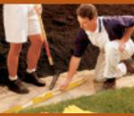
Start by digging a shallow trench 4" deep by 12" wide. Cut through and remove any sod, roots or large rocks. For organic loam soils, dig 4" deeper and add a leveling pad of sand or gravel. Now compact and level the soil to receive the first course of Sedona Stone.
