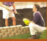
Starting with straight areas first, begin placing the second course. Center each Sedona Stone on the seams of the course below in a running bond pattern as shown. Pull the unit forward until the back lip contacts the unit below. Proceed in a similar manner with all additional layers, backfilling as you go. For drainage behind the wall, use clean gravel or crushed stone as needed.
