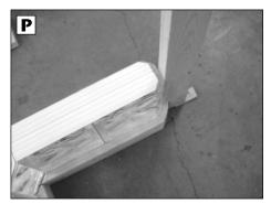
• Repeat this process for every course making sure to install the appropriate vertical spacers at the beginning, at the end and in between the finishing units. Check one final time with a level to confirm that the wall is straight, level and plumb. Use the rubber mallet to help aid in final alignment. Once satisfied, let the sealant dry overnight.
