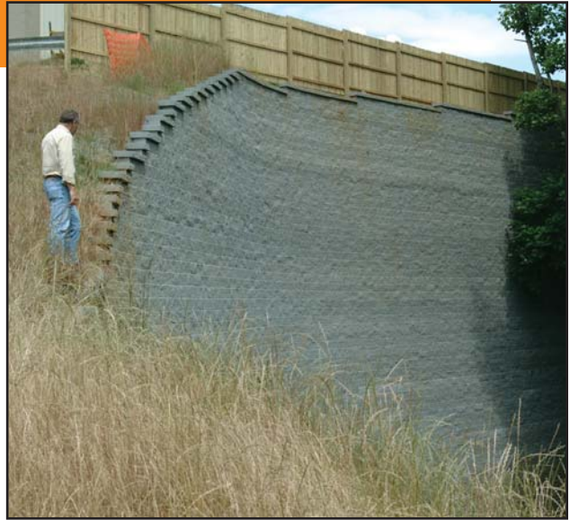
With the help of geosynthetic reinforcement, Square Foot Retaining Walls can be built more than 40 feet tall. — Gainesville, Ga.
