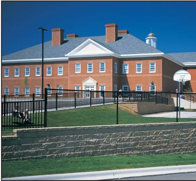
Providence Academy used Square Foot Retaining Walls to create usable space for a playground. – Plymouth, Minn.
