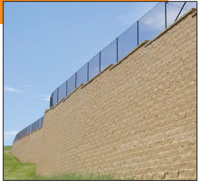
Square Foot Retaining Walls are ideal for D.O.T. projects. – St. Peter, Minn.
